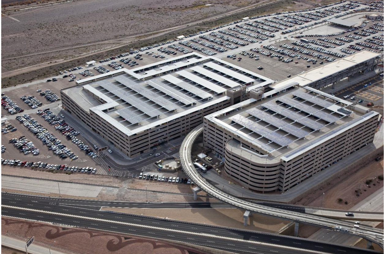
Fig 2. Worley Parsons parking deck solar project
