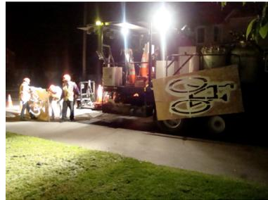
**Figure 4:** The sharrow markings were installed at night to minimize traffic impacts.
